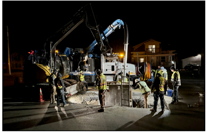
Somers Public Works employees work late into the evening to restore service to residents after a water main break.
