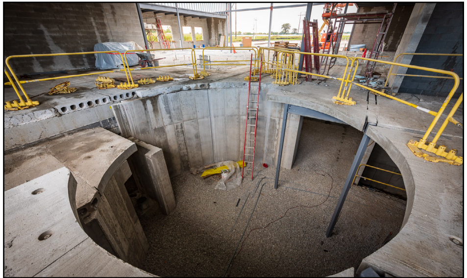
The form for the central stair case at Mission94 has been poured.
