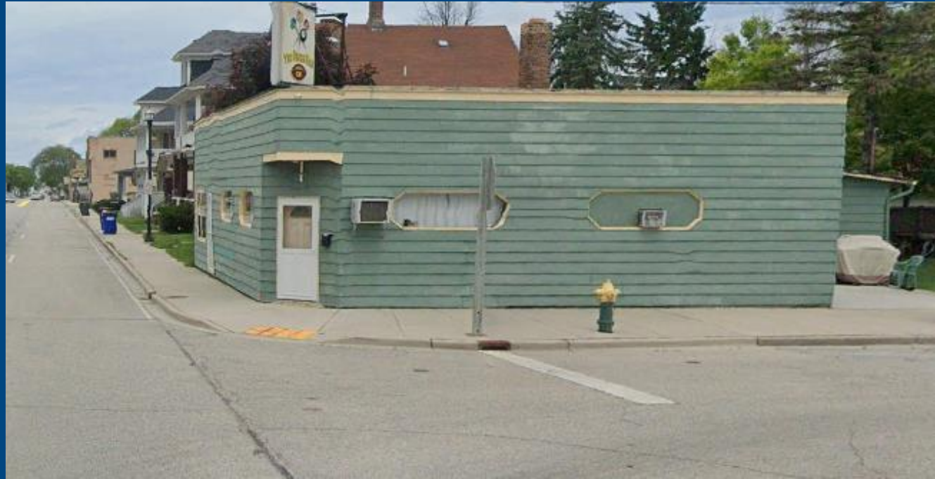
NW quadrant of WIS 32/23 rd St.
