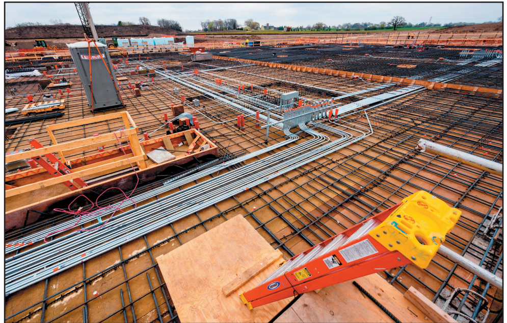
Cables are being run inside the structure of the Pritzker Military Archives Center (top). At right, Village Trustees Jackie Klapproth Nelson and Karl Ostby stand by a mock up of the outside walls of the building which will stand at an outward angle.
